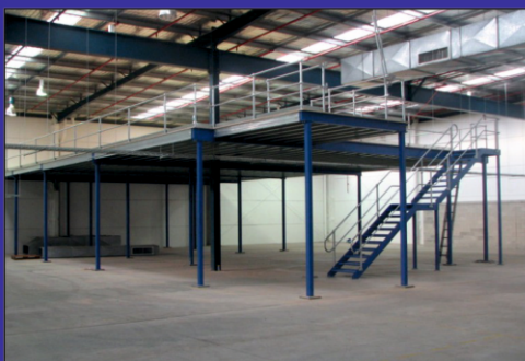
I-BEAM MEZZANINE WAREHOUSE
