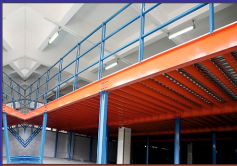
I BEAM MEZZANINE
