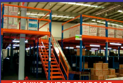
RACKING SLIDER STAIRCASE WAREHOUSE
